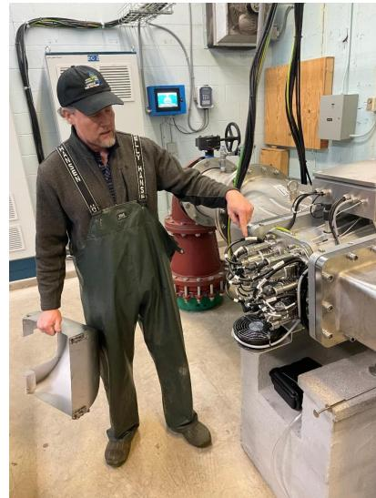
In the picture, Evans points to the array of UV bulbs positioned at the water pass-through. Evans also explained that the device is brand new and the only one in any of the state's hatcheries! Evans can control the device through the illuminated keypad seen on the back wall.
